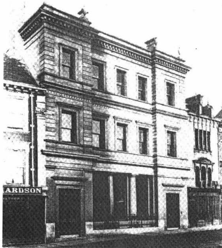
Fig 4: New enlarged Smith's Bank on Rotten Row c1878. Note Fley's Tobacconist still next door but with Mason's Tap House sign removed.
