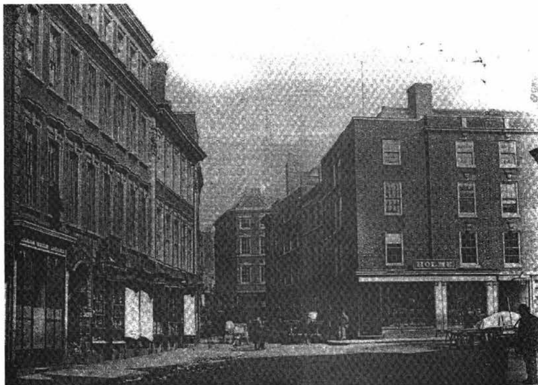
Franceys's House Storer's House Rotten Row The Piazzas Fig 1: From a photograph taken by Richard Keene c1857.
