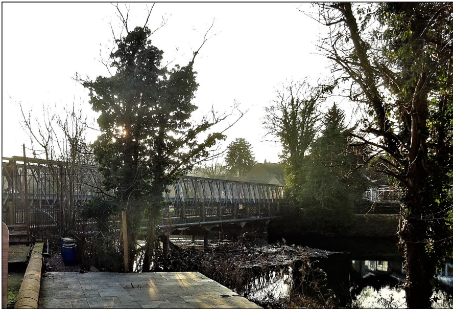
The new footbridge across the Derwent at Darley Abbey Mills, 13 th February 2022 [M. Craven]
