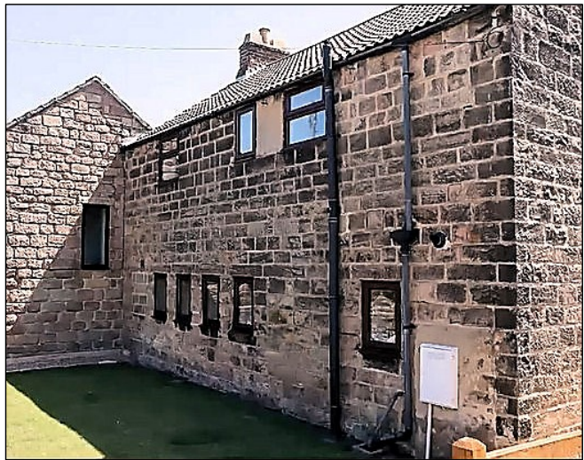
Cottage (much modernised) with original windows blocked off. [Michael Lobb]
