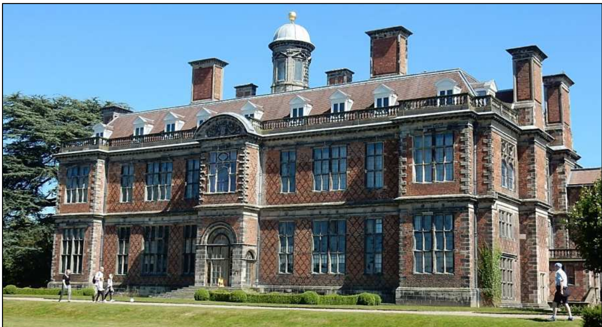
Sudbury Hall, south front with fine diapered brickwork of mid-17 th century date. [R S I Smith]
