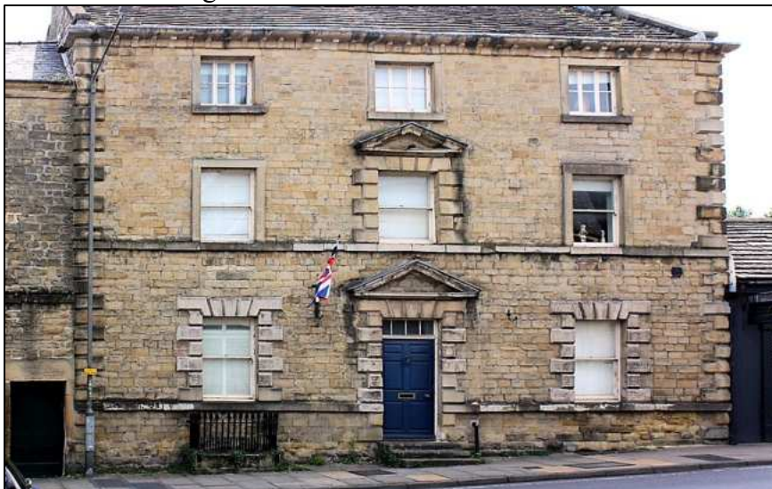
Catcliffe House, Bakewell, with its rusticated window surrounds, busy quoins and wide central bay, suggesting a date nearer to circa 1790-1820, despite the retardataire detailing.
