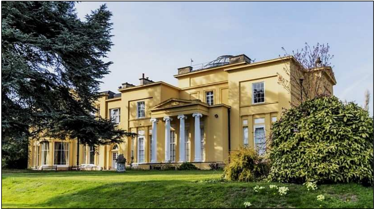
Upton Hall, Nottinghamshire, south front.
