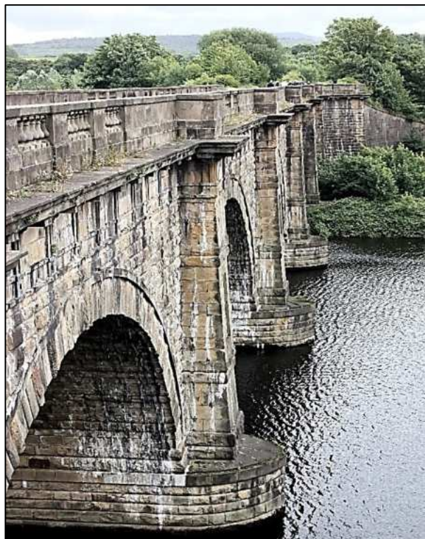
Lancaster: Lune aqueduct, looking north from the Lancaster bank. [David Jones]
